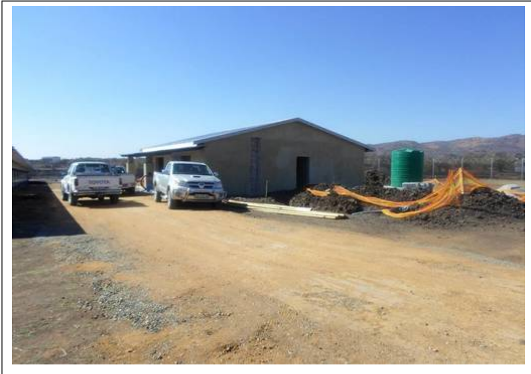
Figure 2: Relay room within the RustMo1 Solar Farm
