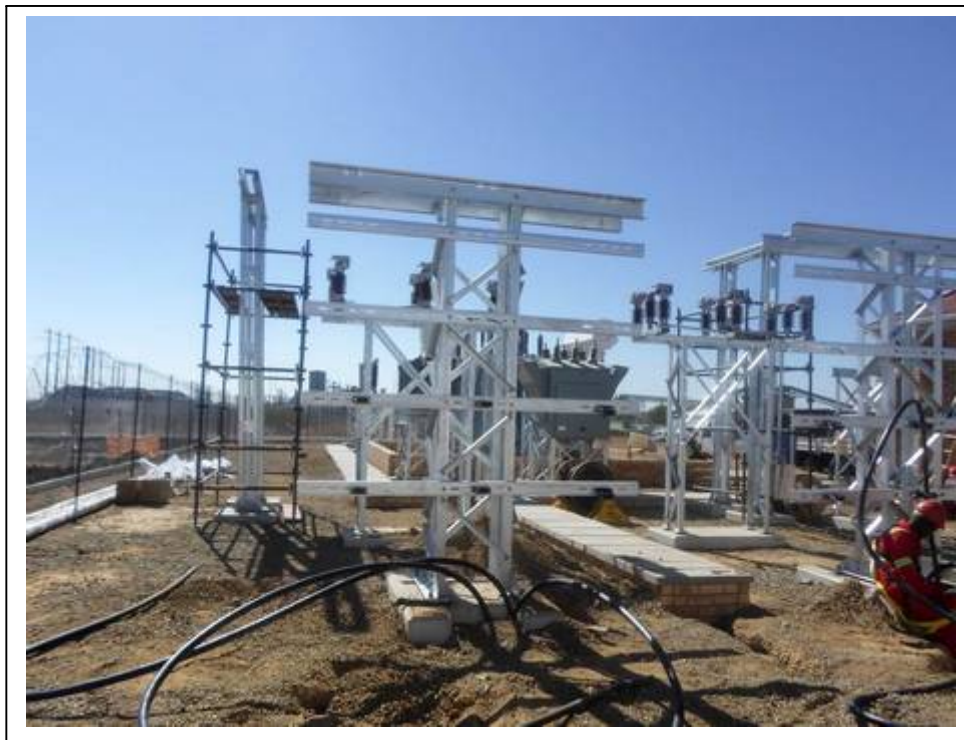
Figure 3: Construction of a 22/88 kV substation on site
